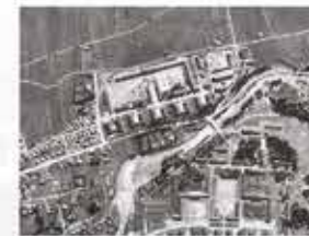
April 19, 1989 plans were finalized for the consolidation of recreation centers. The demolition of buildings on the Sheridan Kaserne began to make room for the new AFRC Resort.
